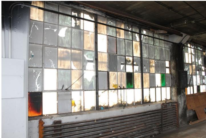
STEEL FIXED PROJECTED WINDOW INTERIOR
