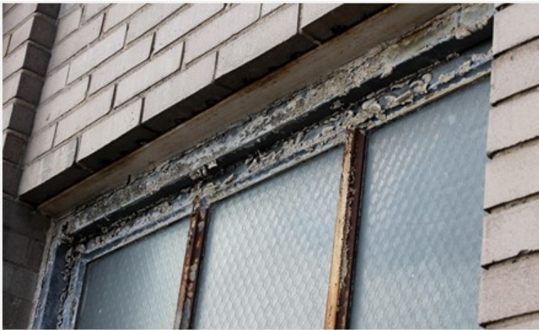
8. Steel Double Hung Window Top Rail, Casing and Muntins
