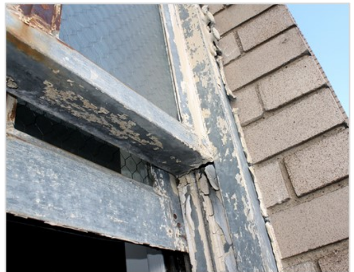
6. Steel Double Hung Upper sash meeting rail and lower sash bottom rail
